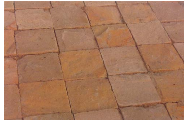
(Fig. 1) Pervious paving allows water to infiltrate into the ground.
