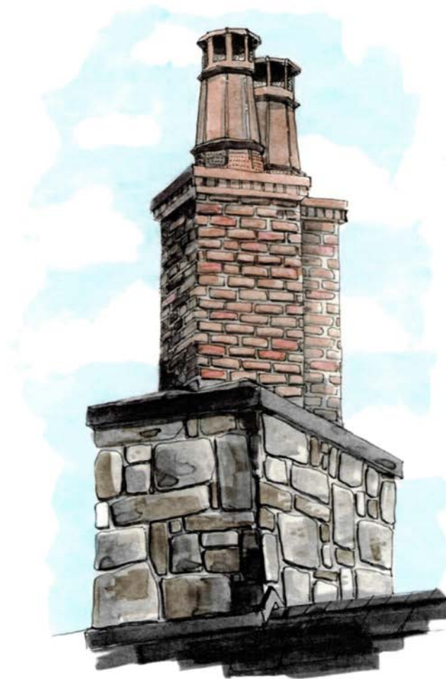
(Fig. 5) Natural Stone and Double-Vented Brick Chimney with Copper Vents
